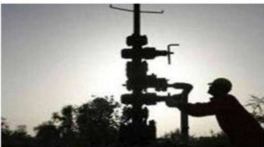
RSGL ready to supply gas to ceramic plants in Ghiloth (Representative image)
